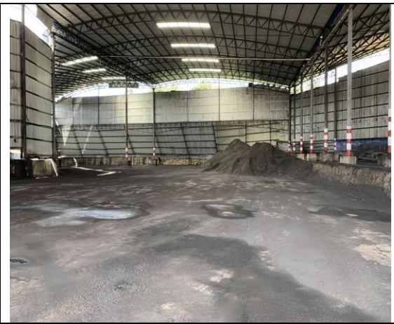
1#钢棚内部现状：堆存少量精煤
