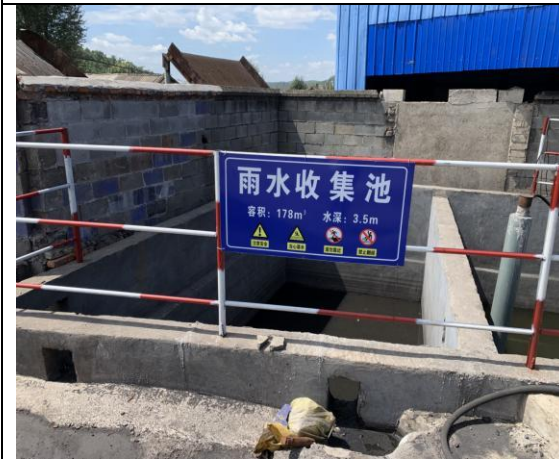
1#钢棚旁雨水收集池现状：容积 178m 3
